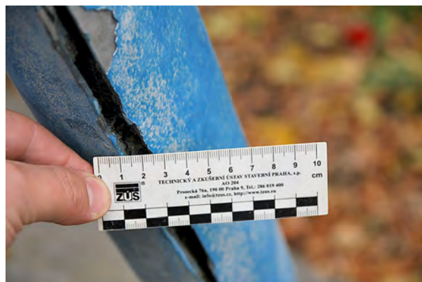
Obr. 11. Široká trhlina v noze sochy Fig. 11. Wide crack in the leg of the statue
